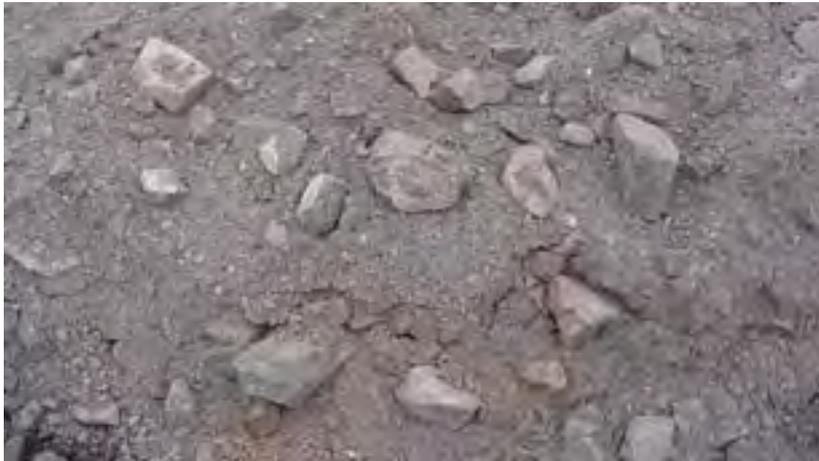
**Figure 1: Coarse Fill before Compaction**
