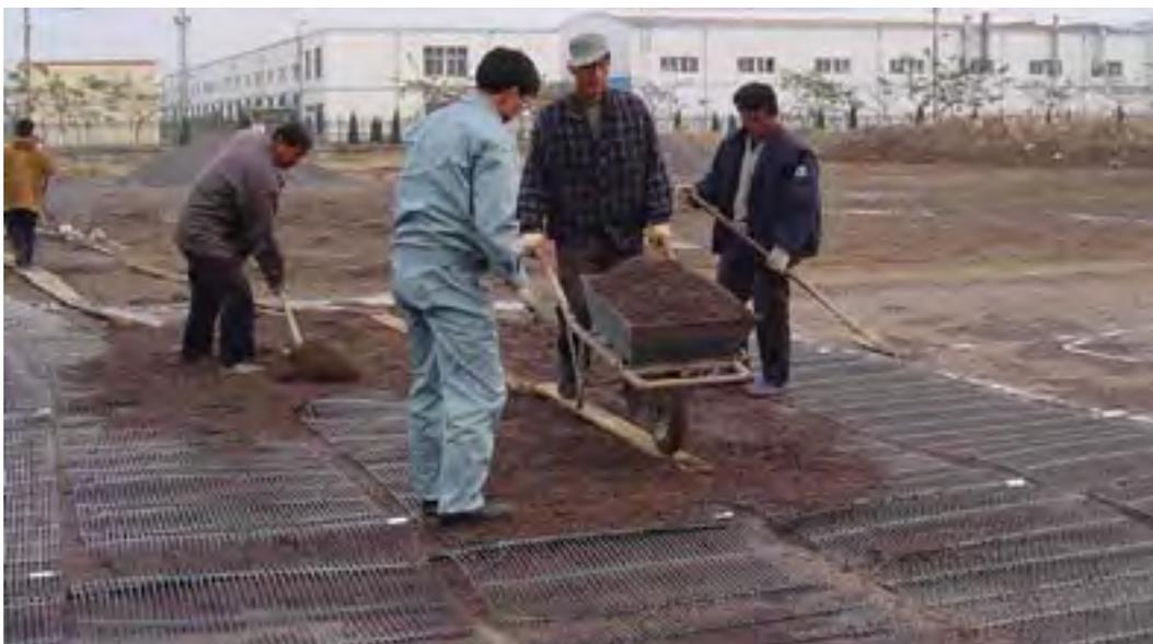
**Figure 4: Placement of Fill on Geogrid Samples**
